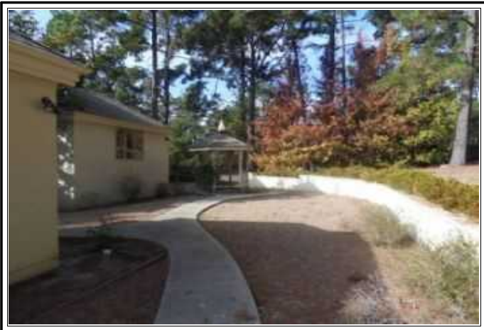
yard area behind garage - deferred maintenance
