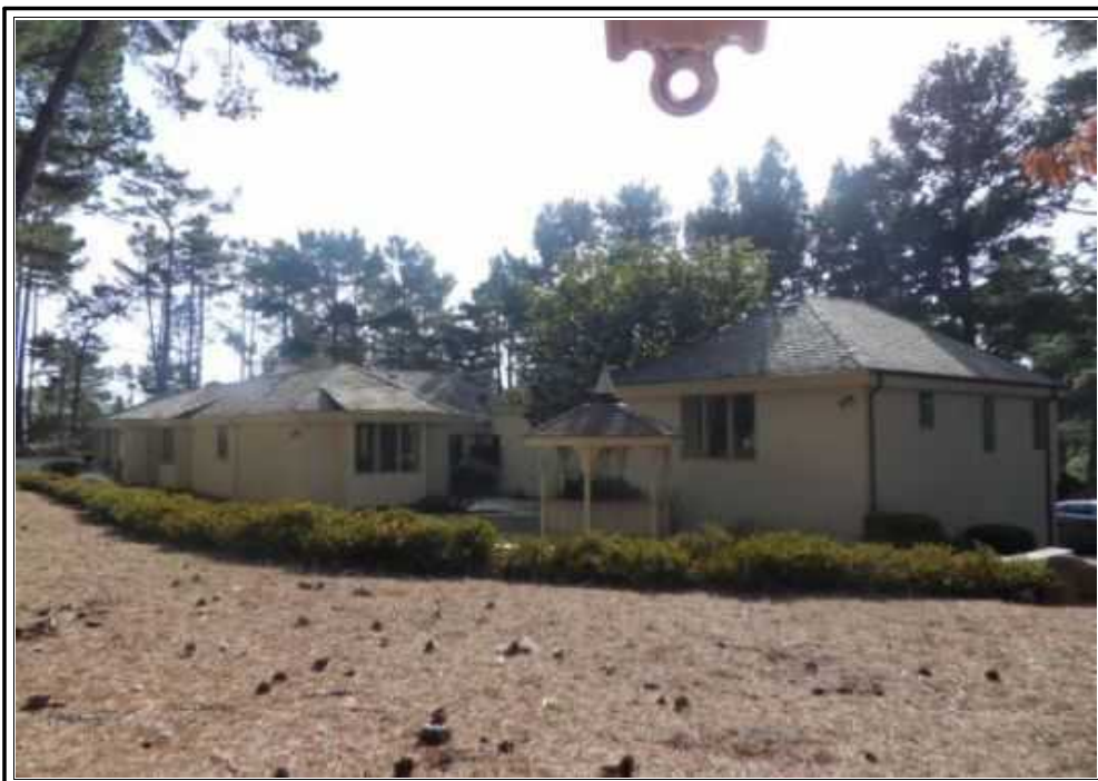
REAR OF SUBJECT PROPERTY
