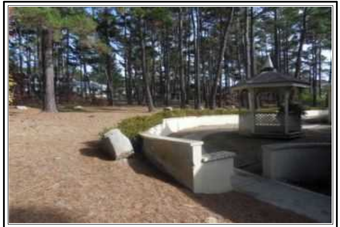
Alternate rear yard north portion deferred maintenance
